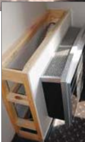
For special rooms, these units had to have mounted louvers to accommodate for ducting.
