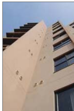
Double core holes from each room keep exteriors clean and classy.
